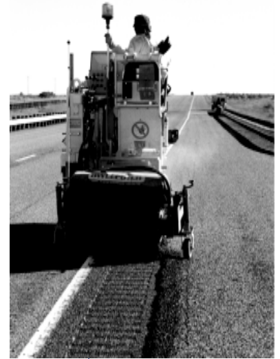
Rumble strips being milled on I-15 near the Montana Border.
